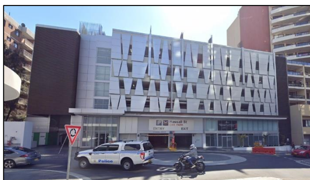
Figure 4: Existing Podium from Hassall Street
